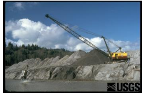
Dredging of the Toutle River after the Mount St. Helens 1980 eruption. Project removed huge volumes of material to prevent river from being choked with sediment.
