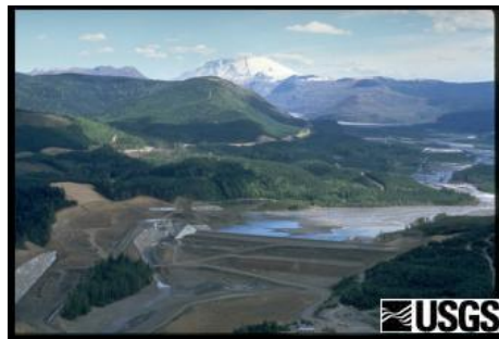
Sediment retention dam on the North Fork Toutle River is designed to help stop downstream movement of sediment near where it begins on Mount St. Helens' debris avalanche deposit.
