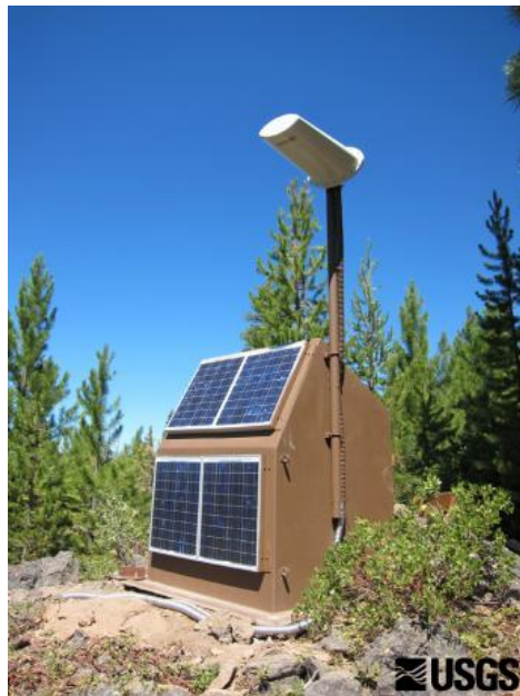
Monitoring enclosure at Newberry volcano, Oregon, with internal monitoring equipment, solar panels, and side-mounted antenna to transmit data.
