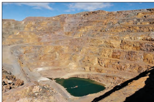
The Mountain Pass mine of Molycorp, Inc., southeastern California, is the only active producer of REEs in the United States (2014). The ore body is a carbonatite intrusion, thought to be the largest REE resource in the United States.
