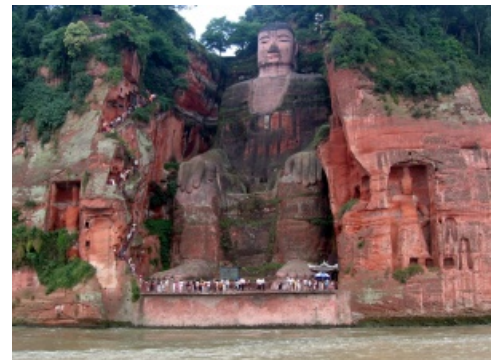
Leshan Buddha in China, 2005, sandstone blackened and corroding from acid rain. Photo by http://commons.wikimedia.org/wiki/File:Leshan_Buddha_Statue_View.JPG Ariel Steiner
