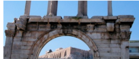
Hadrian's Arch at the Acropolis, Athens, 2005, marble blackened and corroding from acid rain. Photo by Marcok
