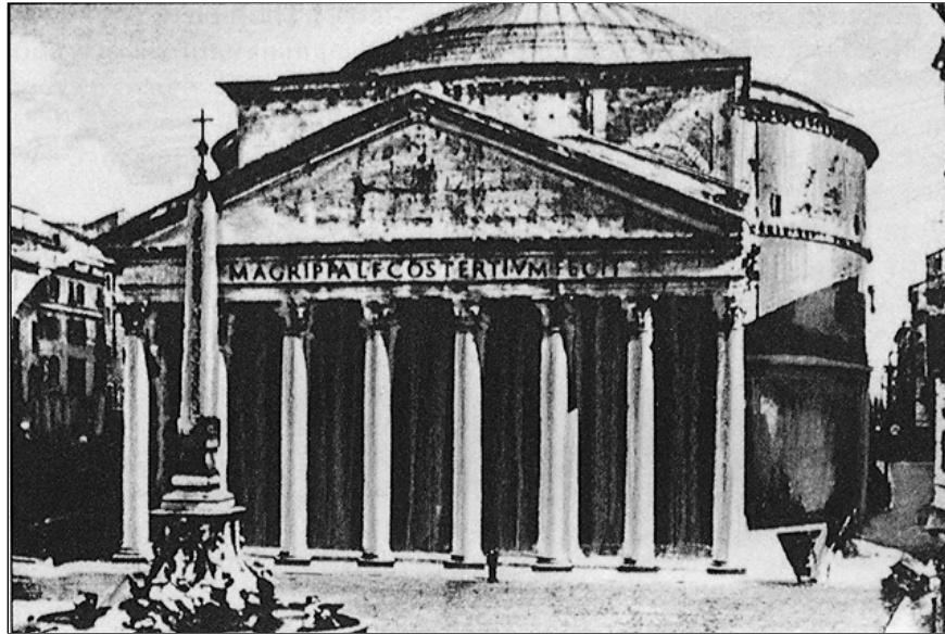
Figure 2. Completed in A.D. 128, the Pantheon of Rome had unreinforced concrete lower walls that were 20-foot-thick. Brick rubble and volcanic stone were used as aggregate. The cement was made from pozzolanic powder which was produced from volcanic ash. The lightest of this pumice was used in the dome which is 142 feet in diameter. The Pantheon is 1,867 years old, and still in fine condition.
